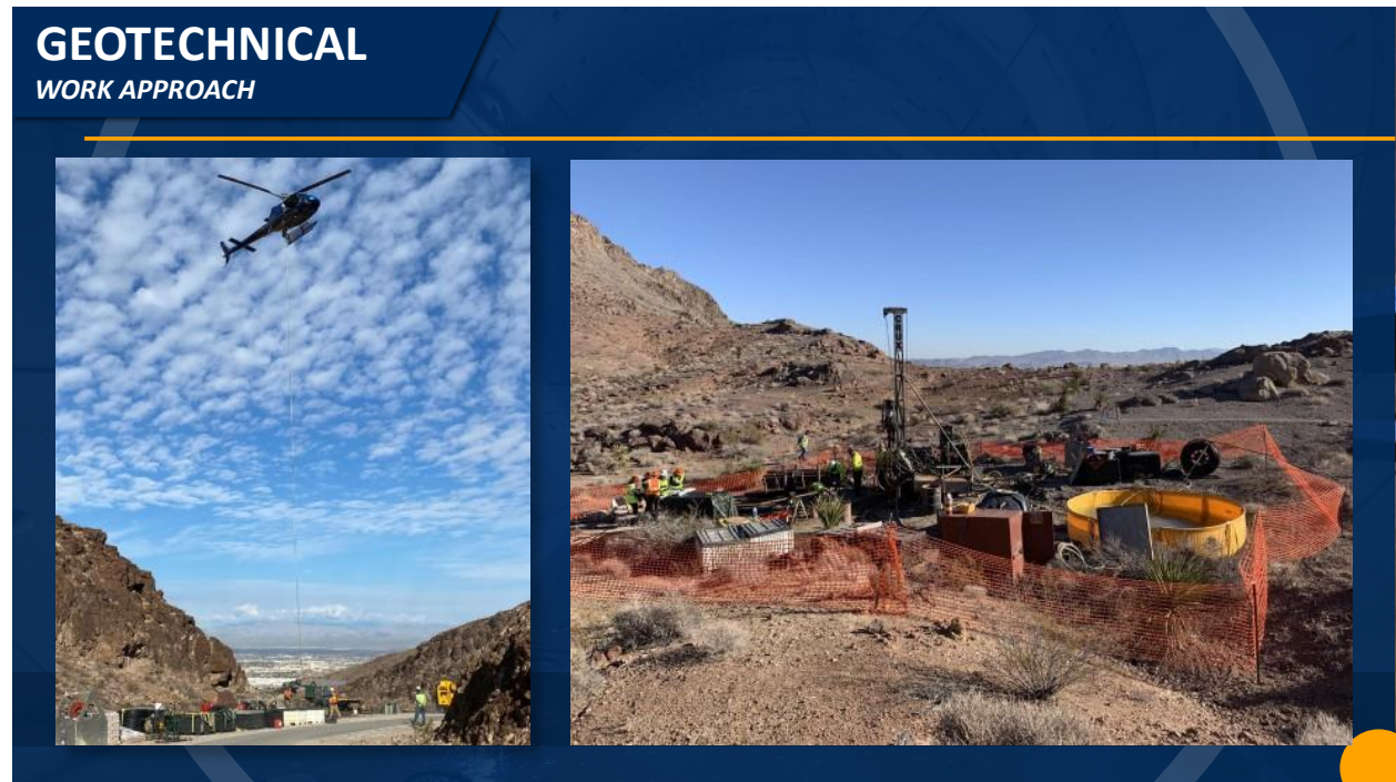
Figure 3: Geotechnical Work Approach
