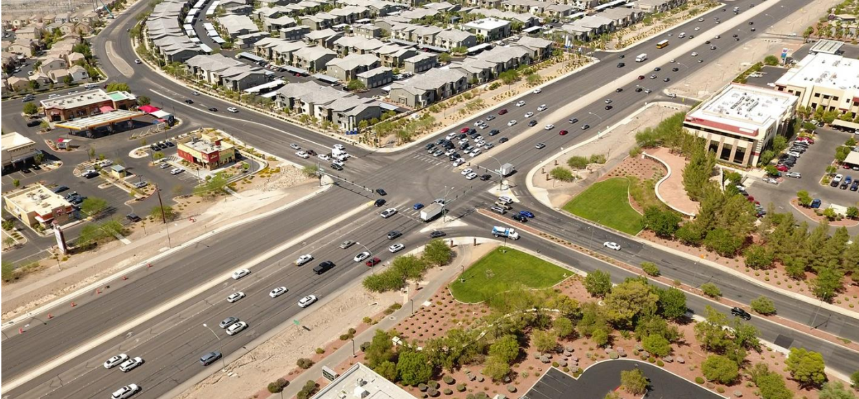
Figure 6: St Rose Parkway Open Trench Construction – Existing Condition
