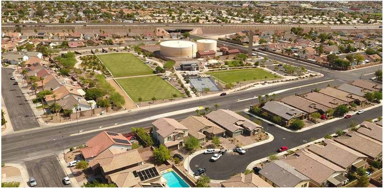
Figure 4: McCullough Vista Park Launch Shaft - Existing Condition
