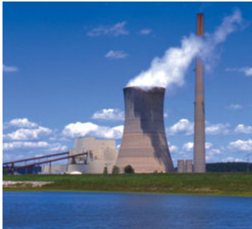
Mountaineer Plant - New Haven, WV
