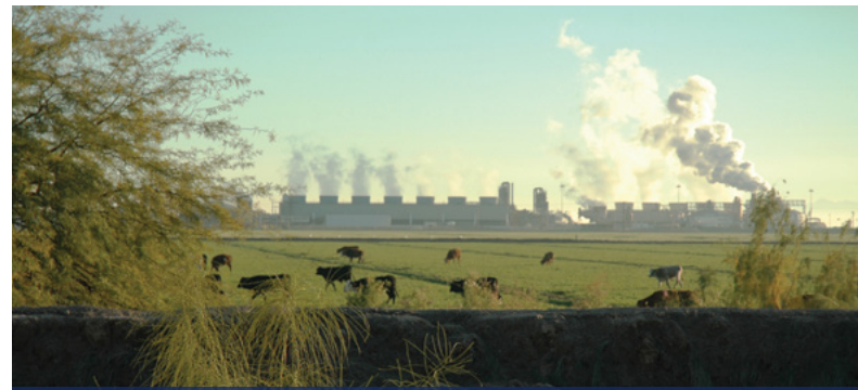
The Hoch and Vulcan geothermal power plants in California coexist amidst the existing land use.
