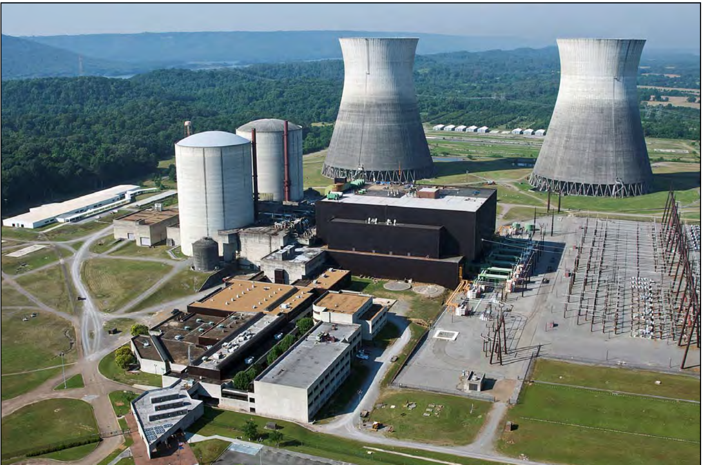
Bellefonte Nuclear Plant Unit 1, Alabama
