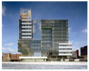
doors and windows are open, and solar panels on the roof, which help to reduce estimated energy costs by almost half. Occupancy sensing dimmers and natural daylighting expect to reduce lighting energy by 45 percent. These and other energy saving strategies earned this building a LEED Platinum rating, the highest LEED rating available.
