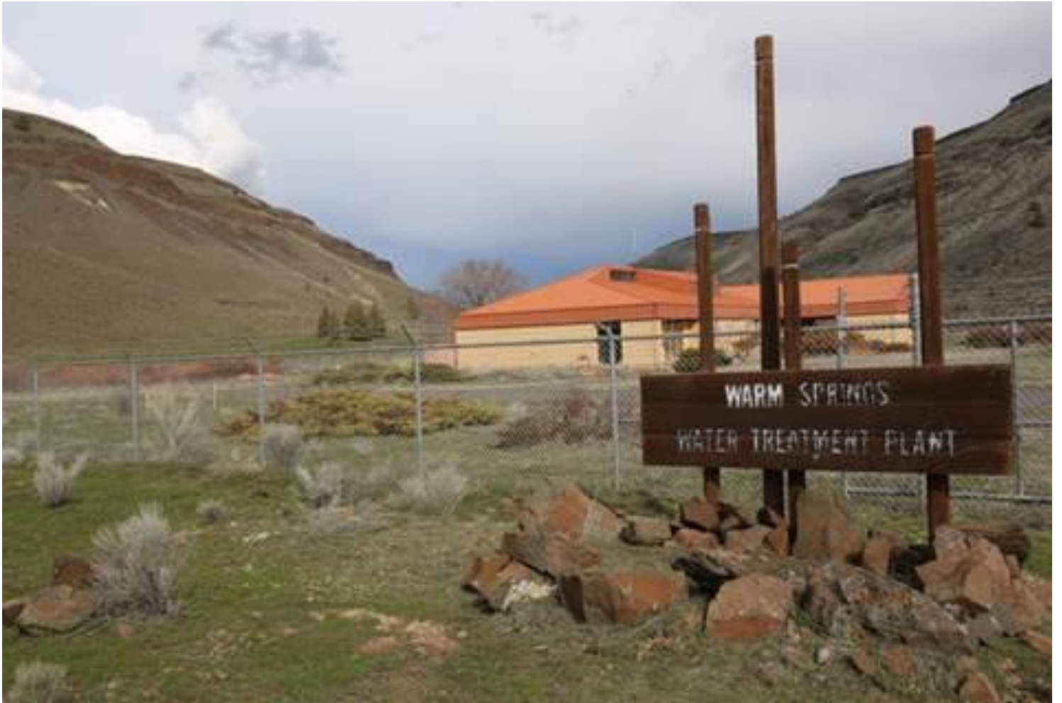
Warm Springs Water Treatment Plant on the Warm Springs Reservation.
